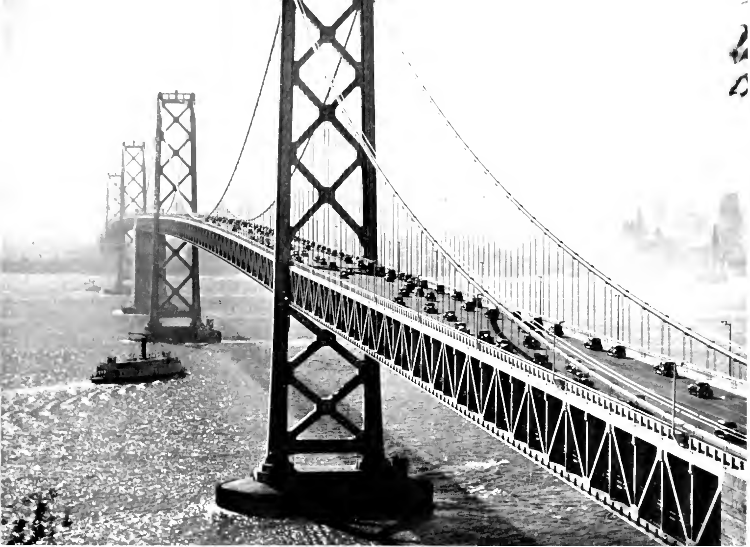
View of San Francisco-Oakland Bay Bridge looking westerly across the structure showing the City of San Francisco in the background
